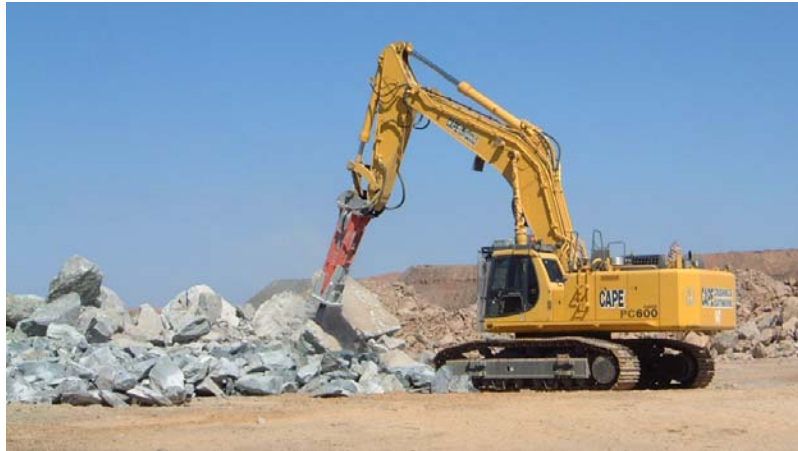
Figure 3 Rockbreaking on the Surface is Restricted to Day Time Only
